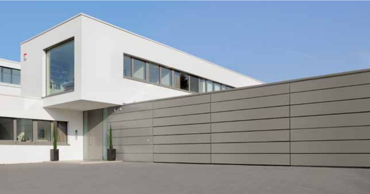
On-site cladding with aluminium compound board
